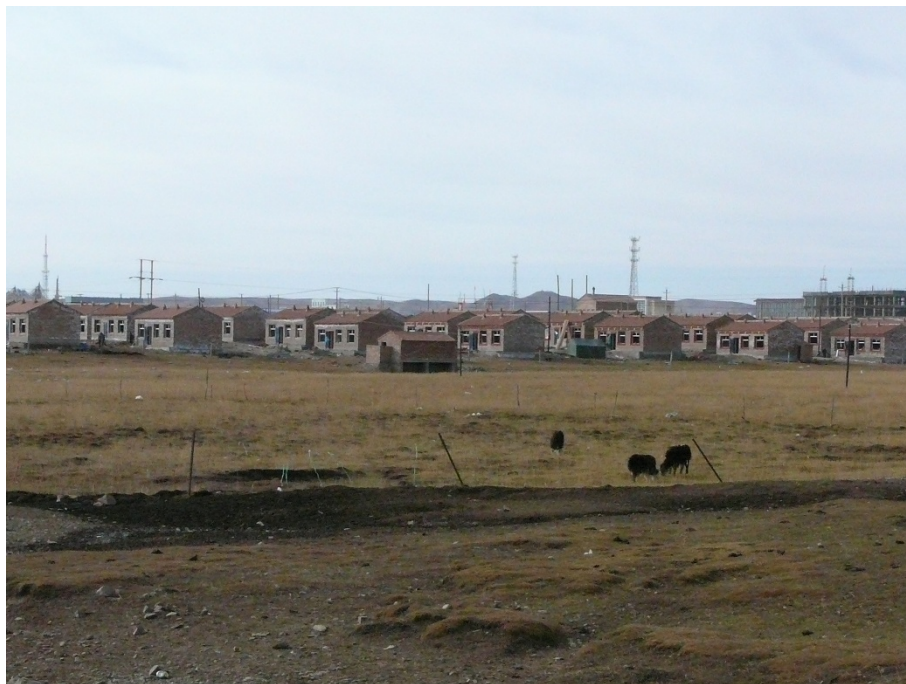
Figure 2 Nomadic settlement project constructions; Zeku County; October 2009.
